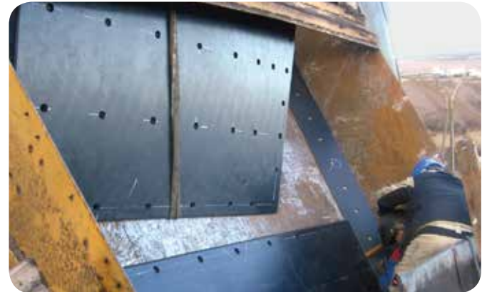
Anti-static: Matrox EX 60 in open-cast mining where explosion risk is high.
